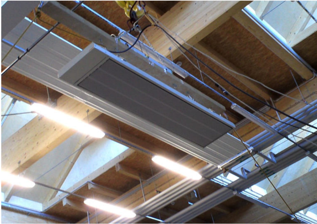
Figure 4-2 Radiant panel Ecosun S+ 30 suspended on auxiliary structure during stabilizing period (front view)
